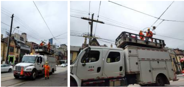
Fig. 1. Testing, measurement, or maintenance of overhead power lines is usually done by a large bucket truck or stage truck to carry workers up to the power line. This operation delays traffic, blocking the road, and putting workers at unnecessary risk.
